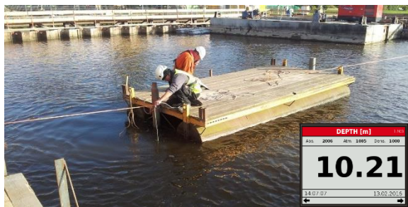
Main: Original visual depth reading on pontoon with lead-line. Insert: New digital readout of depth on MOSS screen
