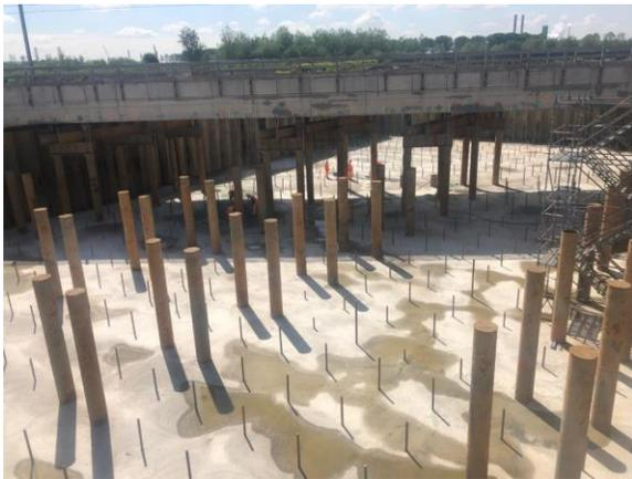
All anchors and piles were measured by divers when excavation-pit was full of water. When water was pumped out a total-station was used for a reference measurement.
