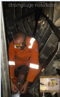
INSTALLATION ON STRUCTURE.
